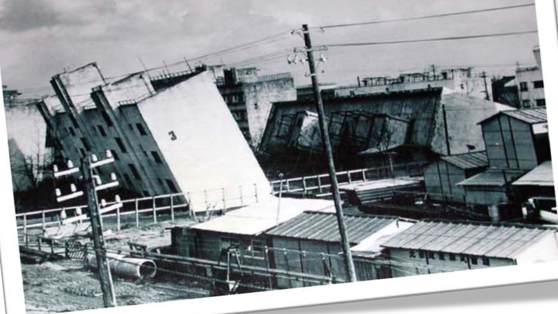
Kawagishi-Cho, Niigata City, Japan 1964: M7.5 Niigata Earthquake
